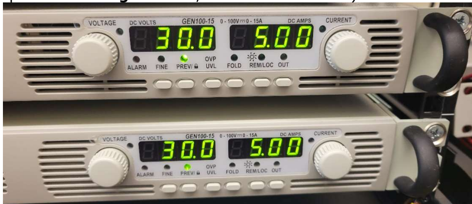
Fig. 8: Checking voltage output setpoint and current limit on the power supplies.
